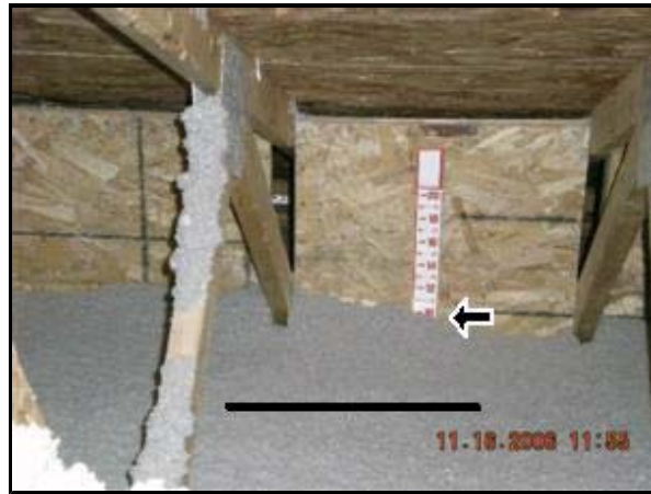
6.0 Picture 2 line is insulation level; arrow is shoved insulation.
